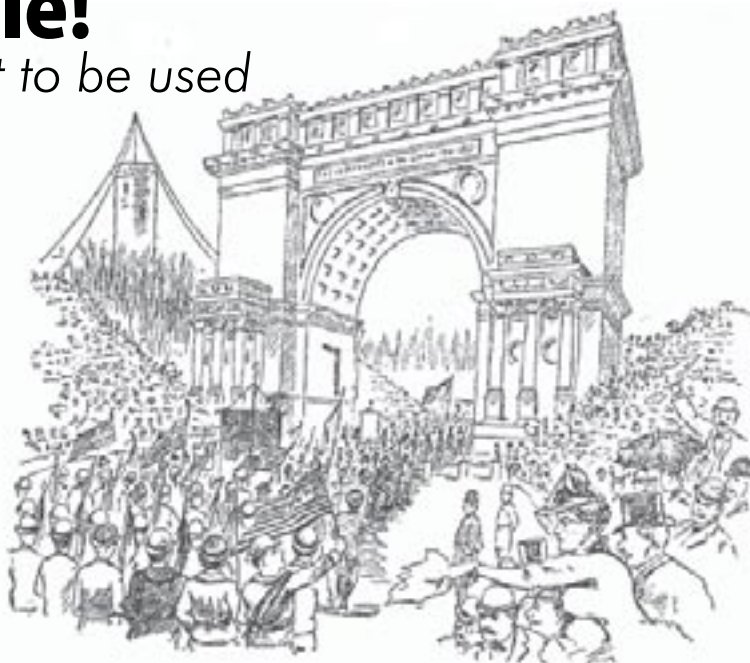
An illustration from the Brooklyn Eagle shows the huge crowd that filled what was then known simply as the Plaza when the Soldiers' and Sailors' Memorial Arch was dedicated on October 21, Columbus Day, 1892.
